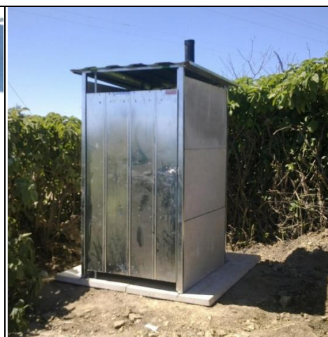
Adopted Rural VIP Pre-Cast Structure
